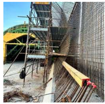
AV/AC Verona-Padova — opere in galleria
